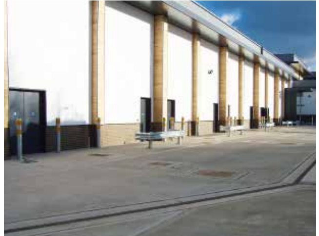
Installation in concrete surface
