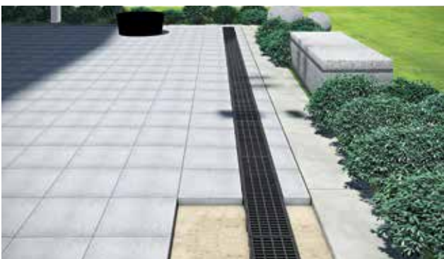
Install surface coating.
