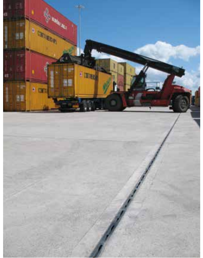
Teesport Container Terminal, Middlesbrough, UK
