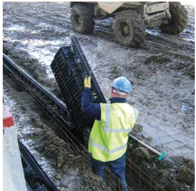
Lightweight elements, installed by one single worker.
