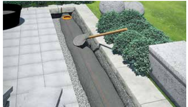
Fill with concrete and compress to foundation.
